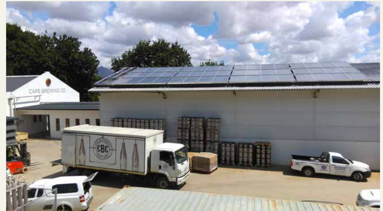
Figure 14: CBC brewery's 120 m 2 flat plate collector array
