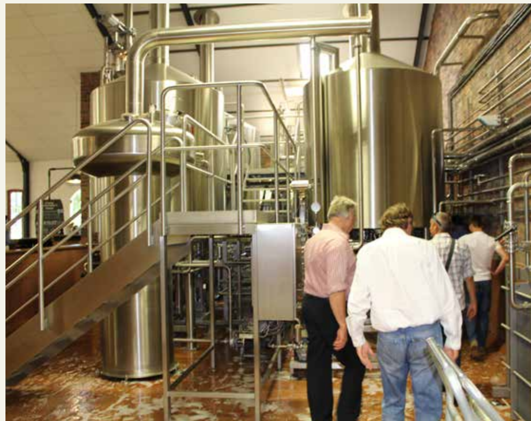
A 120 m 2 flat plate collector feeds into a 10 000 litre storage tank at the Cape Brewing Company. The solar thermal system provides heat for the beer brewing process and hot water for cleaning.
