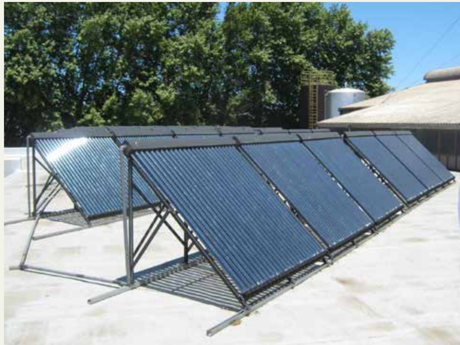
Figure 15: ACA Thread's 156.4m 2 evacuated tube array
